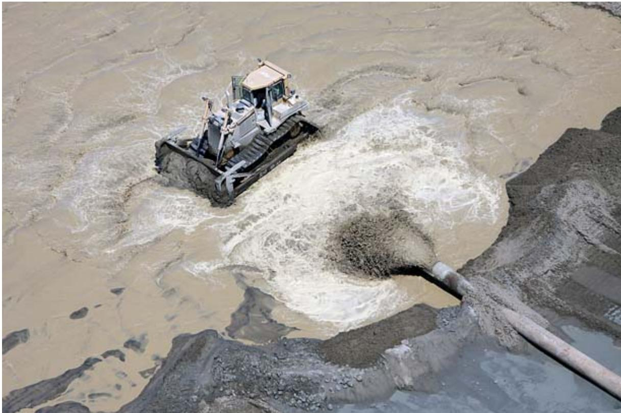
**A key step in the Hamilton Field restoration project: Sediment dredged from the Port of Oakland is pumped onto the marsh plain from the end of a five-mile-long pipeline. Photo: U.S. Army Corps of Engineers, 2008.**
