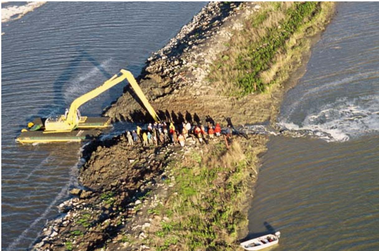
In March 2006, an excavator opened a breach in the levee between former salt pond A19 and Coyote Creek. Photo: Mark Bittner, Pelican Media
